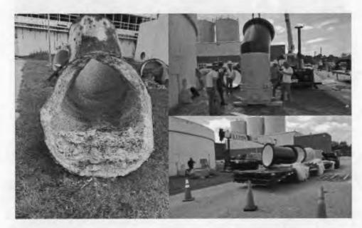
The Contractor has removed old 48" steel pipe and butterfly valve (50+ years old) and is now preparing to install NEW 48" steel pipe and butterfly valve.
