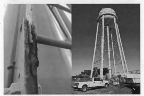
Contractor has repaired and replaced ladder rungs and standoffs that lost their structural integrity (e.g. left picture). The Contractor has also replaced the fall arrest system and installed anti-slip rung tape.
