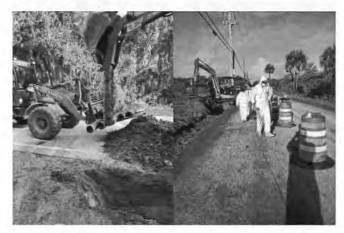
Residents of the Chase Hammock Road segment have been switched over to new 8" DIP water main. The Contractor is currently removing the old Asbestos Concrete water main.
